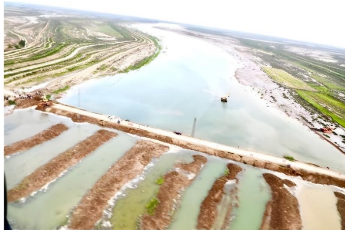
Fig. 2. Flood-control infrastructure in the Al-Musandawq channel.
