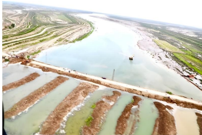
Fig. 2. Flood-control infrastructure in the Al-Musandawq channel.
